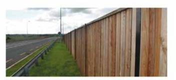
ECC produce components for use in the manufacture of both reflective and absorptive noise barriers. Our reflective acoustic fencing is designed to reflect noise waves with up to 28dB reduction in noise. Alternatively, we supply timber for absorptive acoustic fencing which is covered with a protective membrane on one side of the boards to further reduce noise by an average of 4dB.
